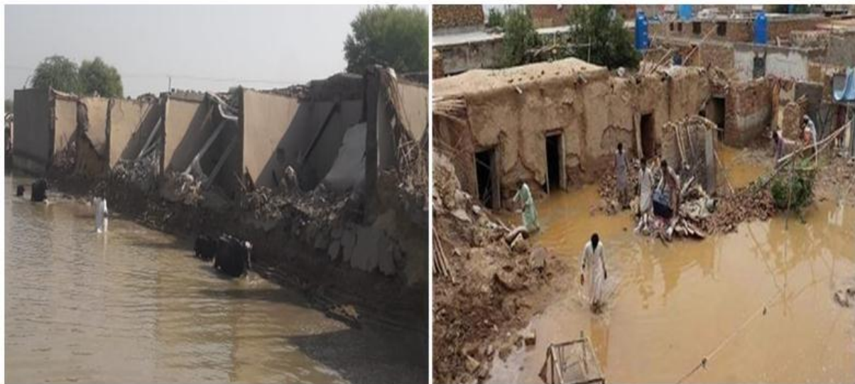
Figure 2: Destruction of homes & Infrastructure due to flood in D.I.Khan
