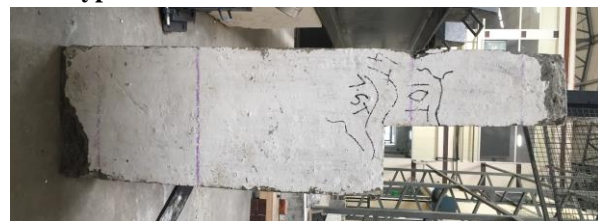
Fig.6(c). Crack pattern for Type 3 SCC
