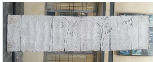
Fig. 6(d). Crack pattern for Conventional Beam
