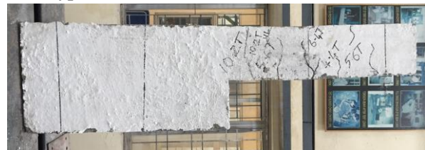
Fig. 6(b). Crack pattern for Type 2 SCC
