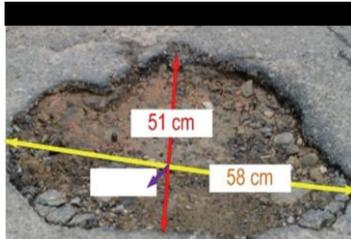
Figure 6: Potholes with height and depth
